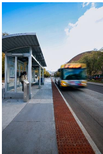
4th and University, Fall. Source Alliant Engineering
