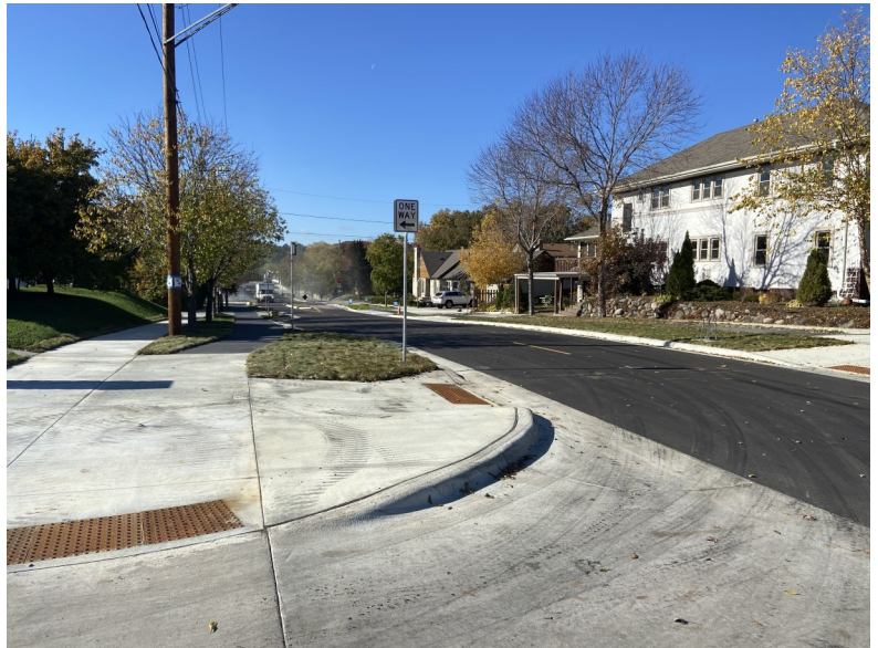
Bump out on Plymouth Avenue, Minneapolis. Image courtesy of SRF
