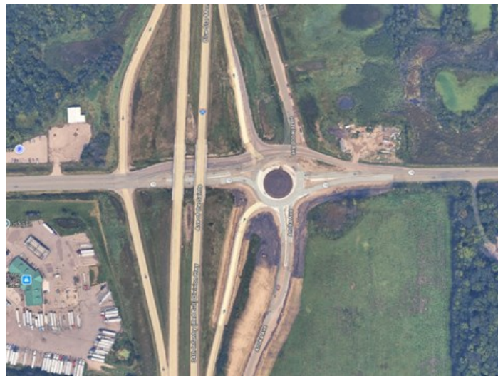
Aerial Image of Stage 2A of the project. Image courtesy of Google Imagery.
