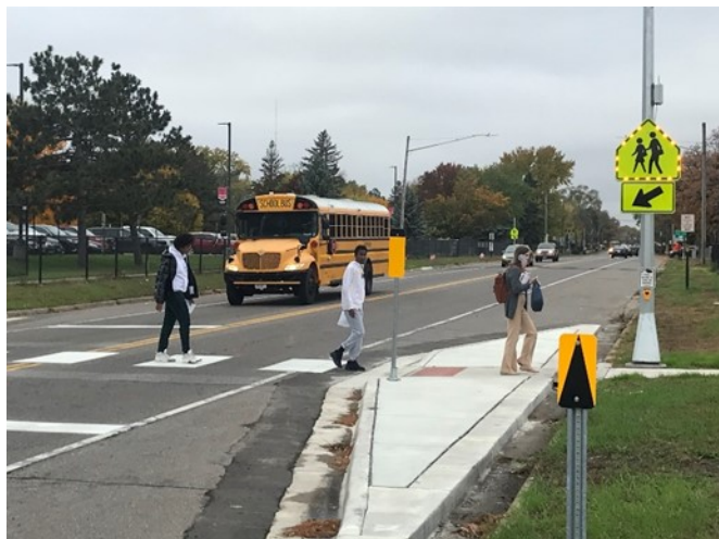
Curb extensions and RRFBs complement reduced speed limits in school zones to improve yielding and compliance for drivers.
