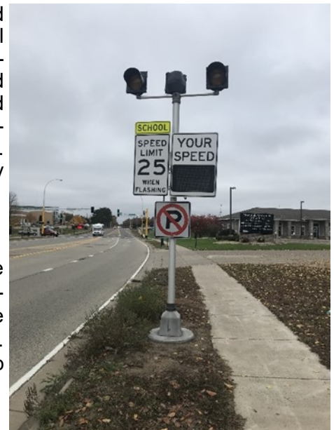
Additional countermeasures such as flashing beacons and other design solutions further increase compliance of reduced speeds in school zones during school arrival and dismissal. This is an example of a Flashing System and School Zone Speed Limit at Coon Rapids High School.
