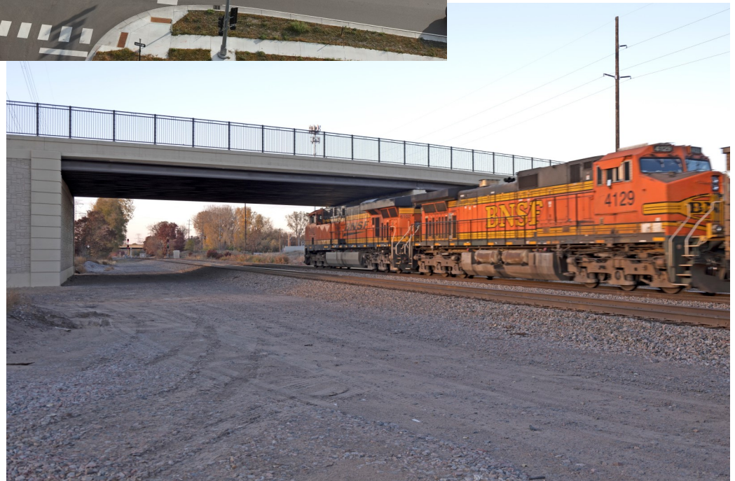
The structure type is prestressed concrete beams with a pier in the BNSF Railway right-of-way. The bridge layout is compatible with BNSF Railway's future plans and operations.
