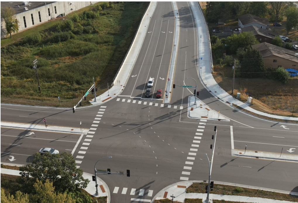
The East River Road and Foley Boulevard intersection was relocated approximately 400 feet to the northwest. Traffic signals were installed at East River Road, Norway Street/Metro Transit, and Coon Rapids Boulevard.
