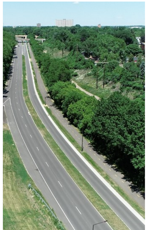
Left: Construction photo of Ayd Mill Corridor facing south taken after paving shared-use trail.
