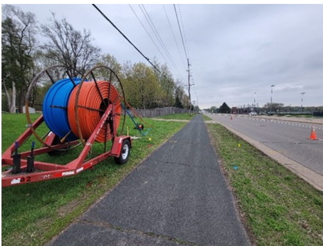
Left Image: Fiber Conduit Installation in Eden Prairie. Right Image: Handhole/Fiber Installation in Edina.
