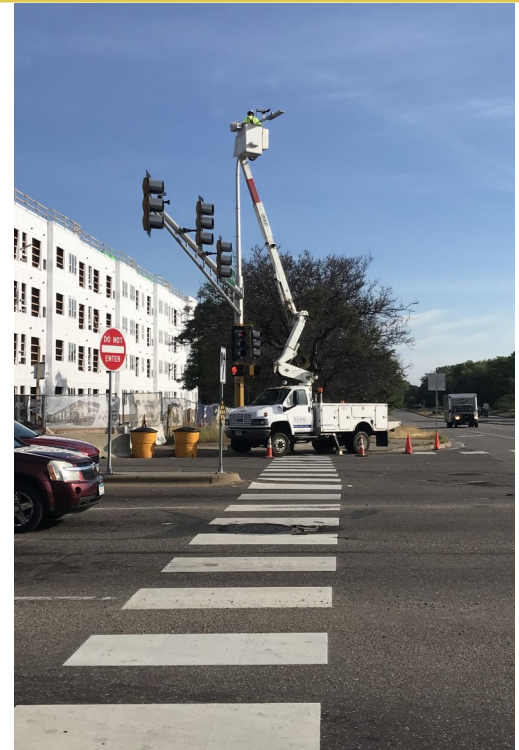
Testing Device Installation
