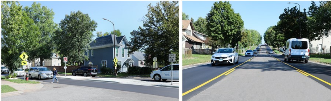
Figure 4: Examples of recently completed 4-lane to 3-lane conversions completed by Alliant for Ramsey County
