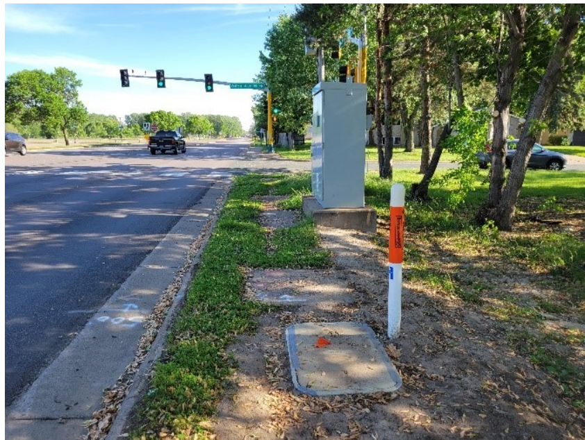
Handhole and Fiber Marker Installation in Brooklyn Park, Minnesota
