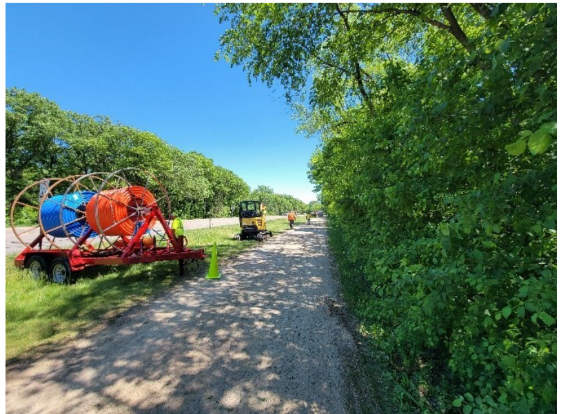
Fiber conduit installation in Minnetonka, Minnesota
